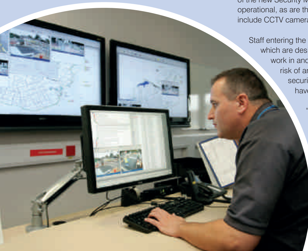
An operator observes CCTV footage in the new Security Monitoring Centre.
